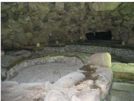
Made of split-face blocks in 1925, the house exhibits a grotto, parapet, four Jacuzzis, and a pool. But with 55 documented leaks, Playboy Enterprises knew there was a serious problem. Using thermal imaging, the sources of the leaks were identified and a solution was sought.
