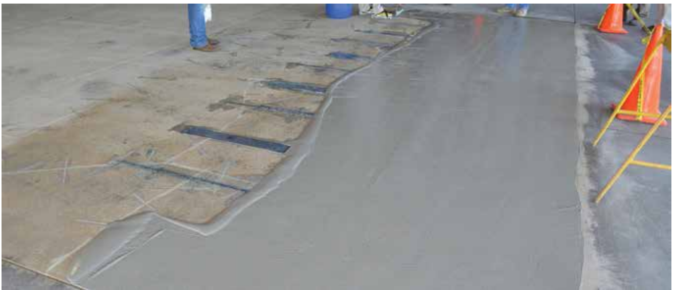
Cementitious Overlay Installation Over Strapping and Stapling Repair
