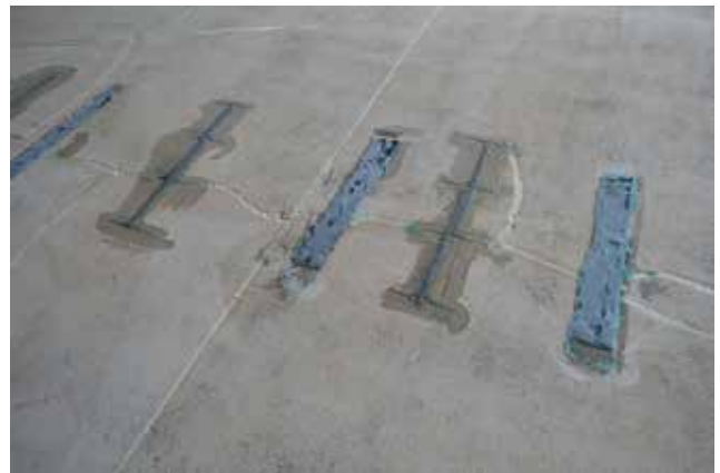
Carbon Fiber Strapping and Stapling Repair
