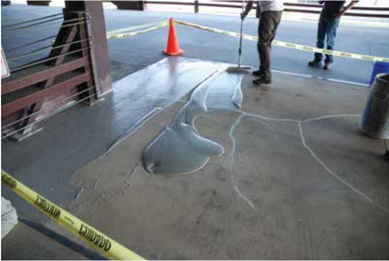
Applying Cementitious Overlay
